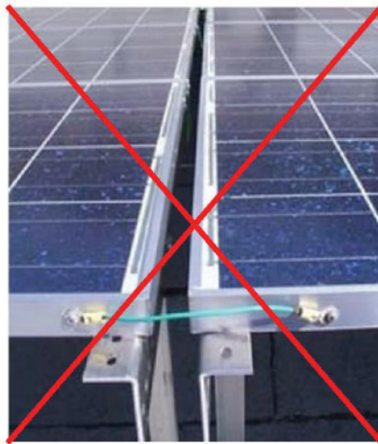
Photo B3 – Example of acceptable connection of bonding conductor
