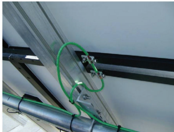
Photo B3 – Example of acceptable connection of bonding conductor
